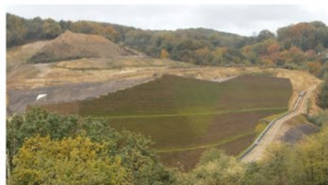
Ecological walls in front of the plot, facing the facility. Compacted and horizontally reinforced embankments with geogrids.
