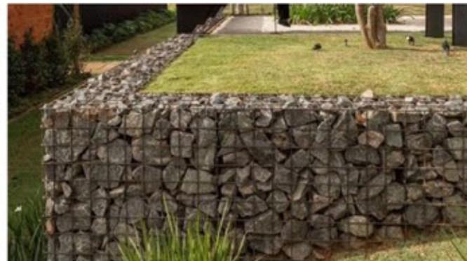
Retaining walls for private gardens with gabions.
